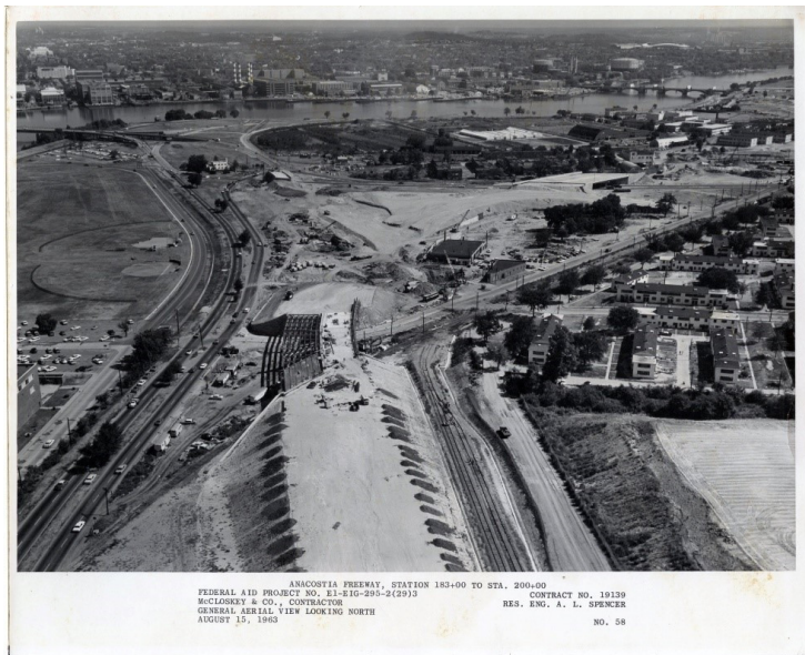
Anacostia Freeway (I-295), under construction (August 15, 1963)
